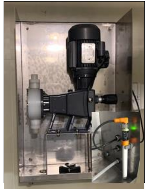
Figure 4: Sulphuric acid pump
