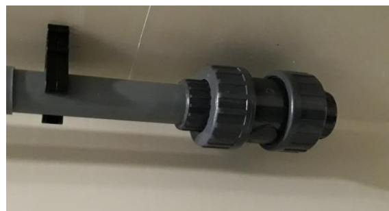
Figure 4: Safety valve
